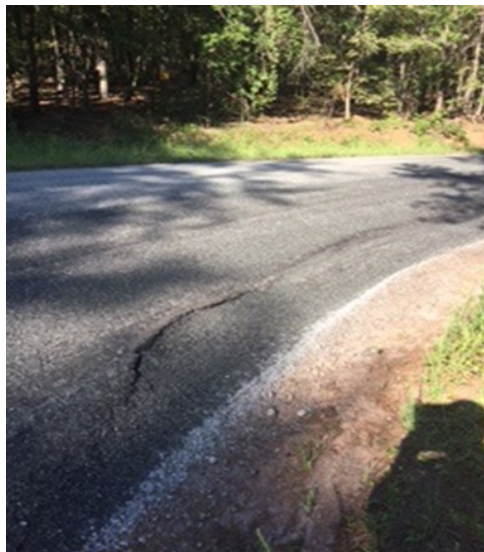
Figure 1-5. Example of poor shoulder work.
