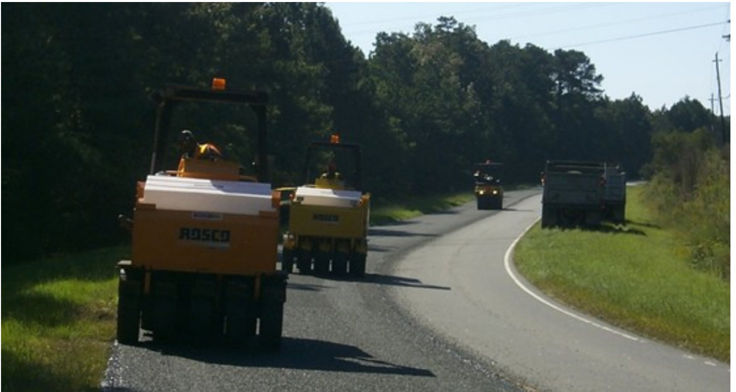
Figure 9-2. Two pneumatic tire rollers followed by a static steel wheel roller.
