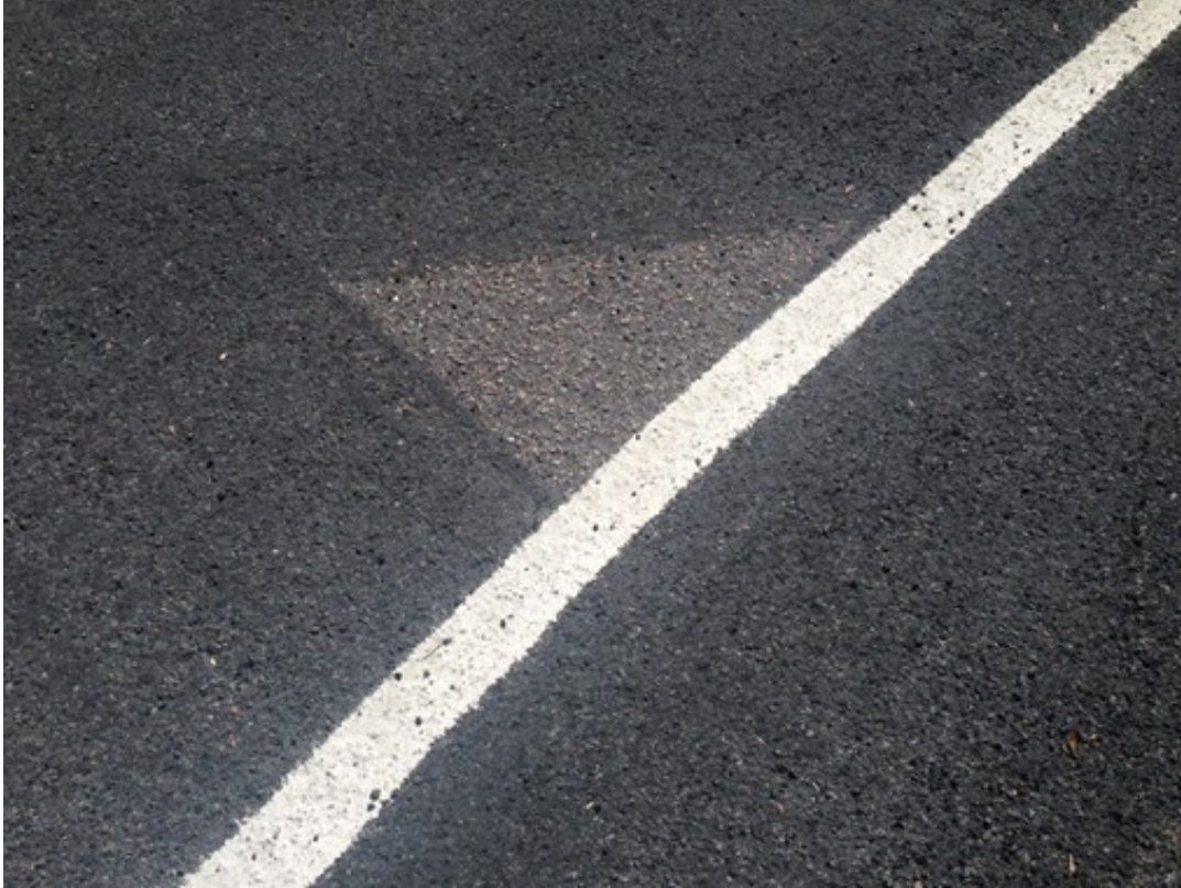
Figure 11-1. Example of insufficient emulsion.
