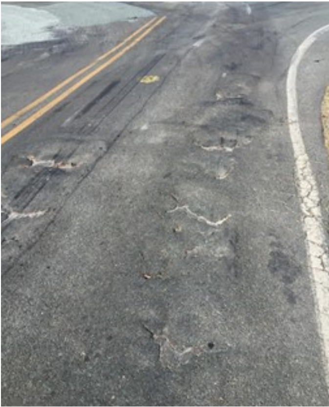
Figure 1-3. Example of severe alligator cracking.
