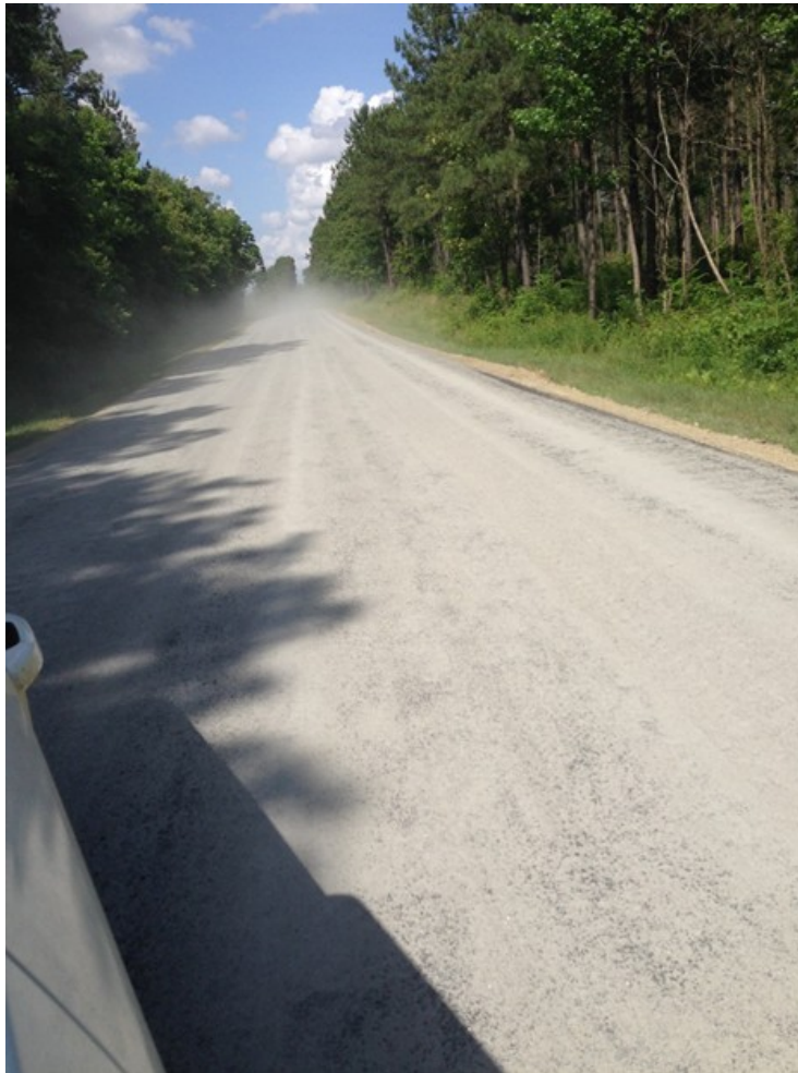
Figure 11-4. Example of excessive aggregate.
