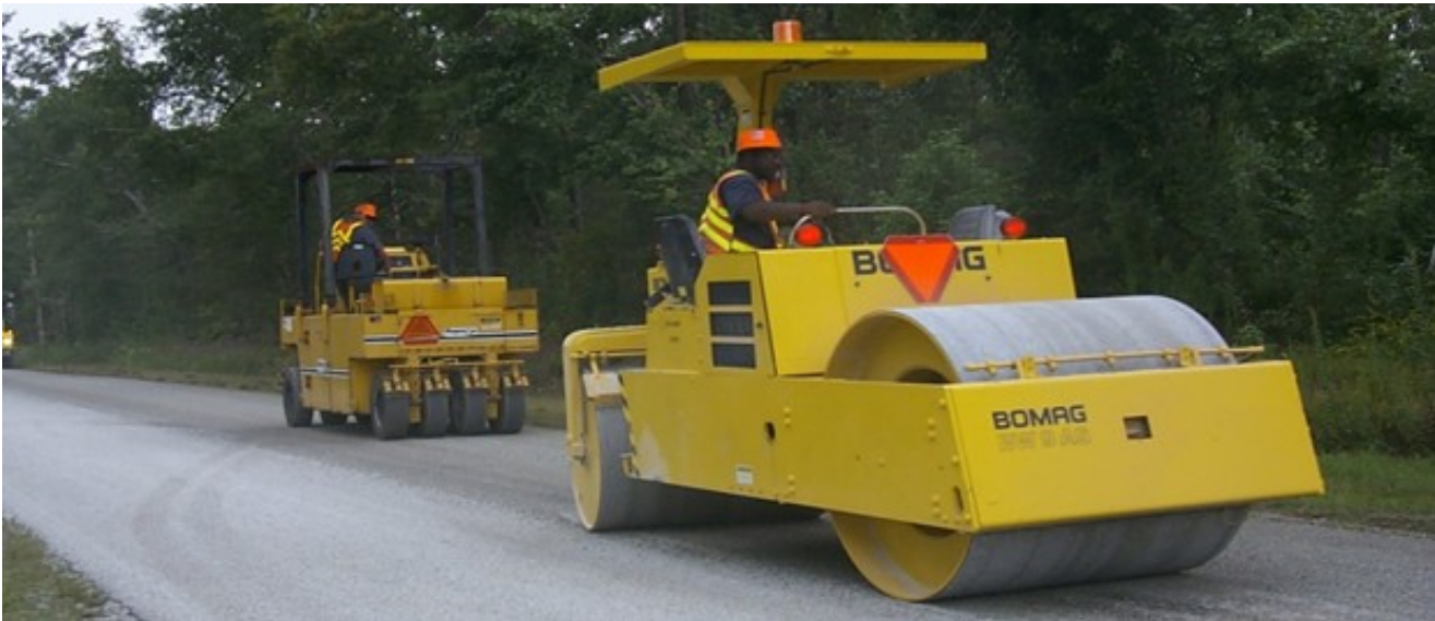
Figure 3-5. Pneumatic tire roller (Background) being followed by static steel wheel roller (Foreground).
