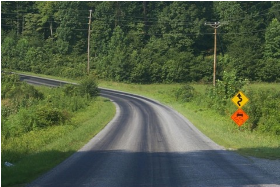
Figure 10-1. Example of a bleeding road.
