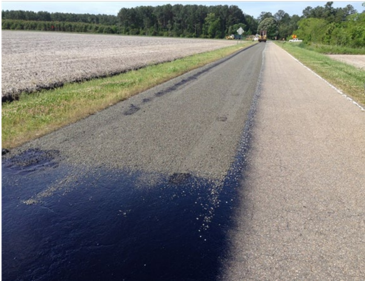
Figure 11-3. Example of insufficient aggregate.
