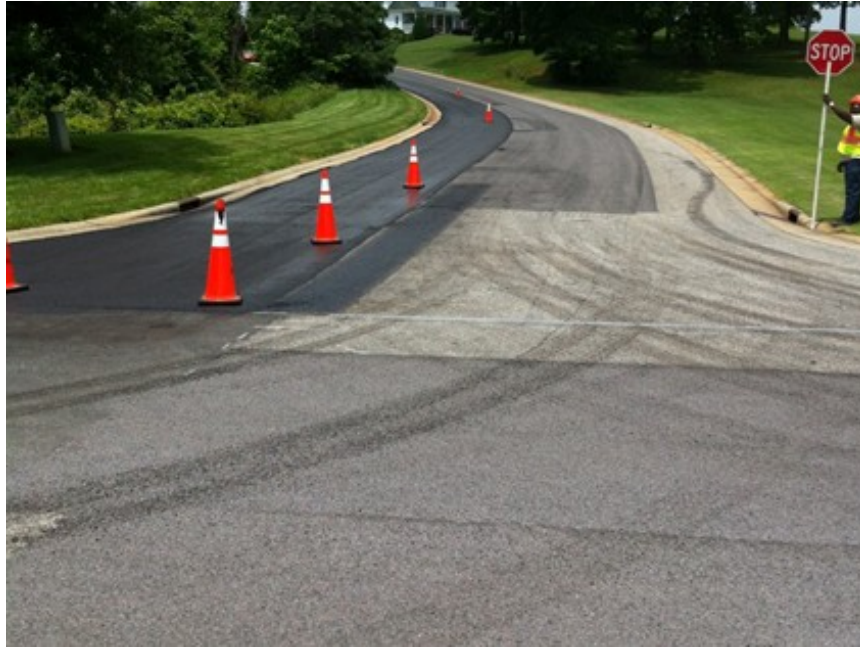
Figure 10-2. Example of an oxidized road.
