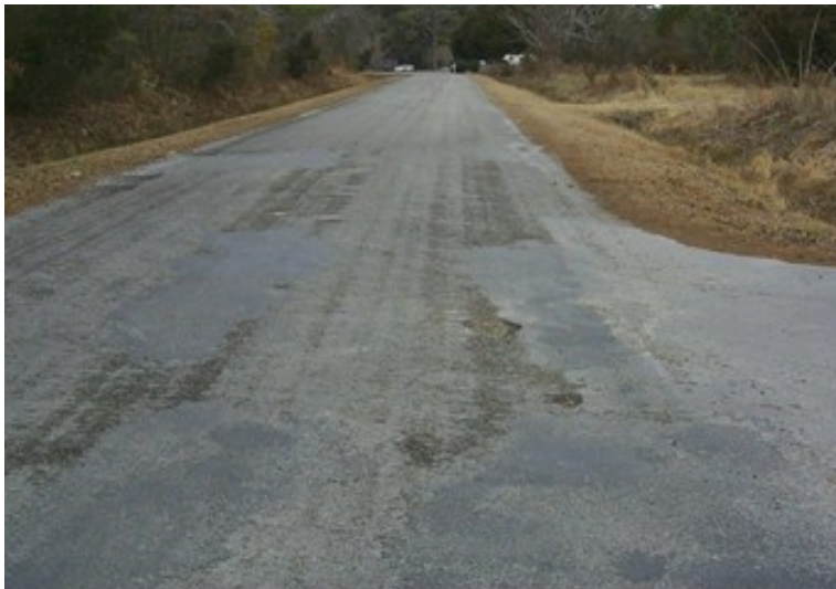
Figure 1-2. Example of rutting.
