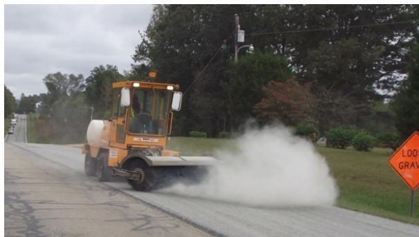
Figure 3-7. Mechanical broom in use.
