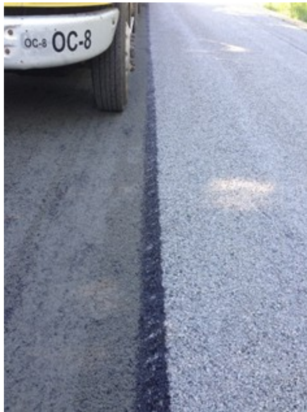
Figure 12-1. Example of centerline tie strip or longitudinal joints.
