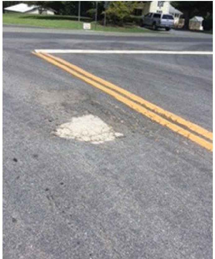
Figure 1-4. Example of a concrete patch.
