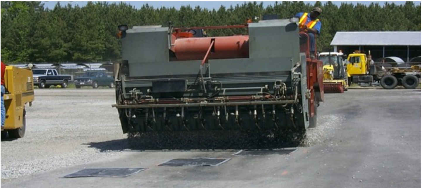
Figure 3-10. Calibration of the stone spreader.
