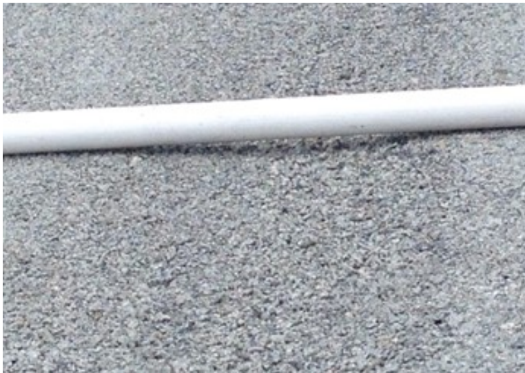
Figure 1-2. Example of rutting.
