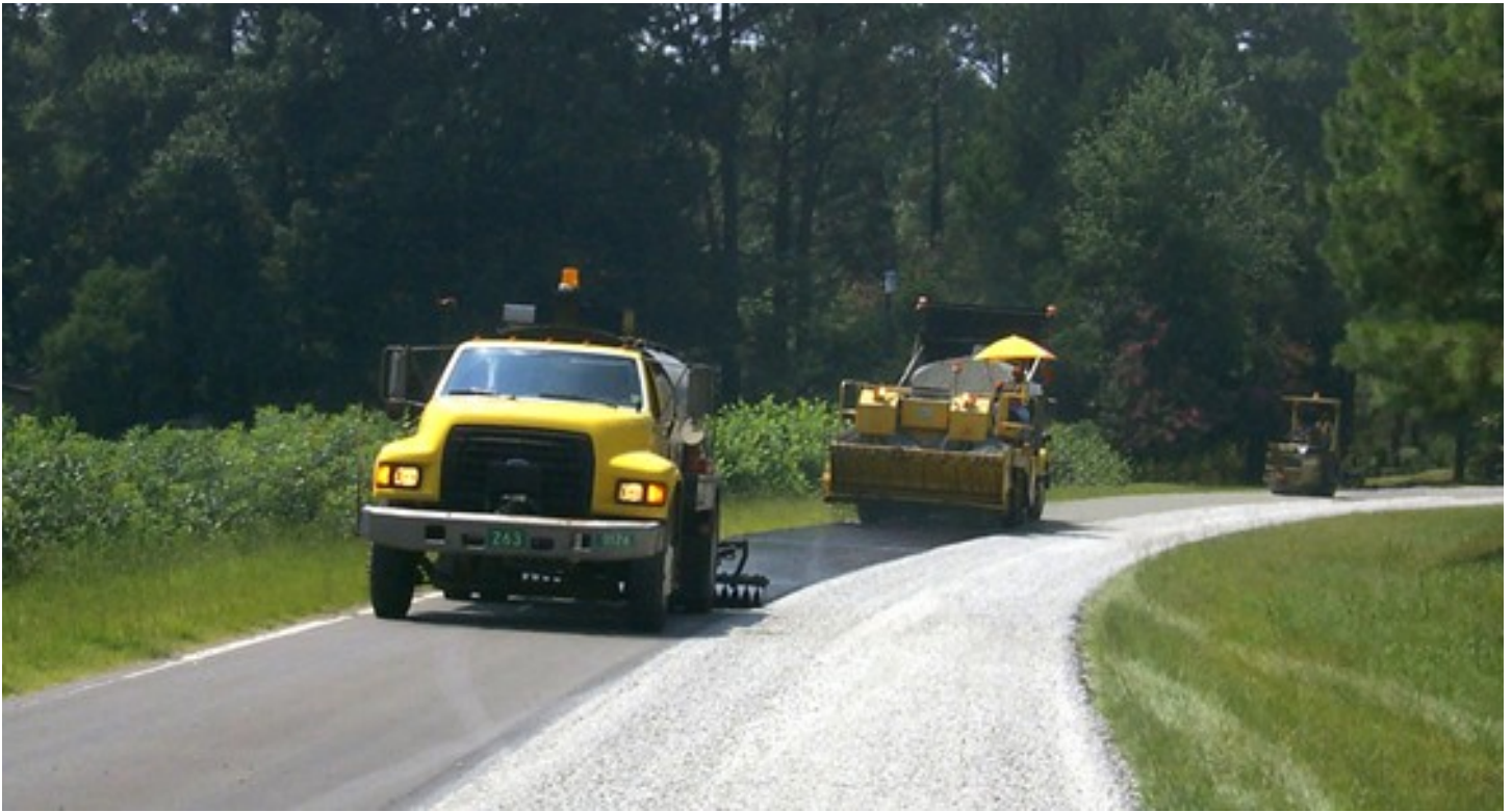
Figure 9-1. Asphalt distributor followed by the stone spreader and roller.
