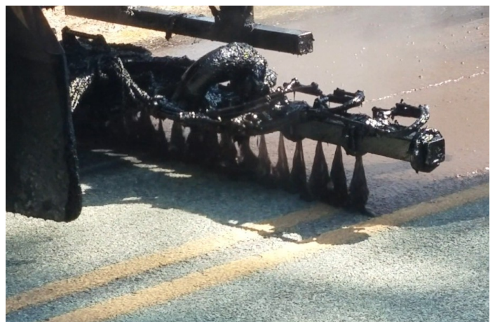
Figure 3-2. Asphalt distributor in use.
