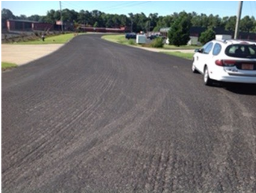
Figure 11-2. Example of excessive emulsion.
