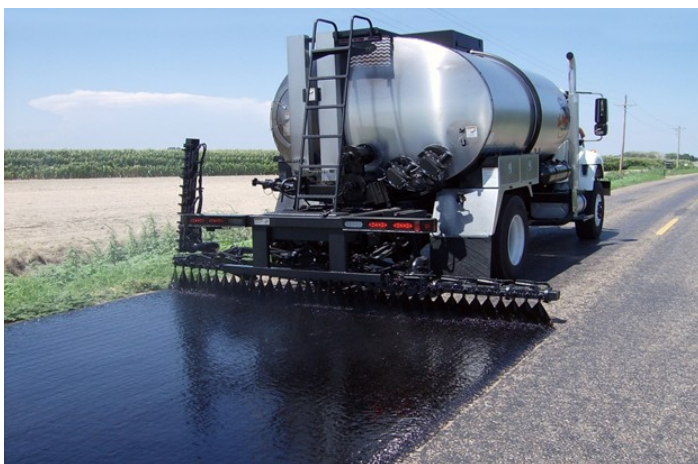
Figure 3-1. Asphalt distributor operating at the proper spray bar height to apply double coverage, courtesy of E.D. Etnyre & Company.
