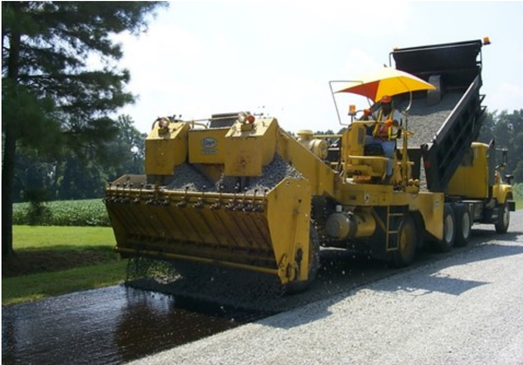
Figure 3-3. Stone spreader attached to dump truck.
